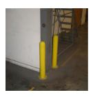
DSB surface mount bollards are constructed from heavy gauge tubing and installed around any fixture that requires superior protection from forklift and pallet jack impact.
